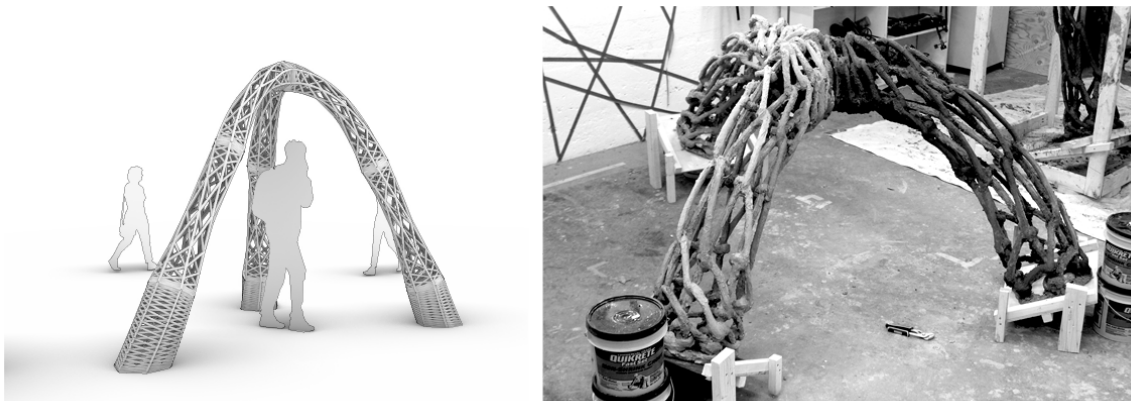
Figure 4. "Augmented Weave: Urban Net." Overall target geometry and in-progress assembly of woven cementitious composite building components.
